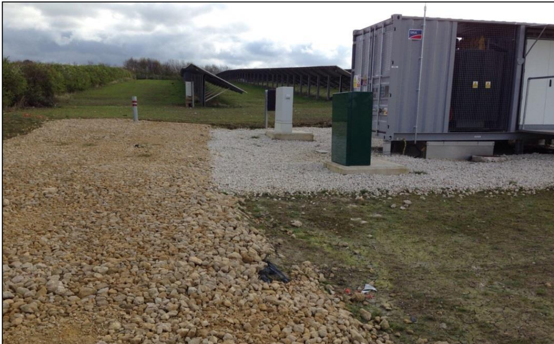
Plate 14: Typical Type 2 Aggregate at Solar Farm 34
